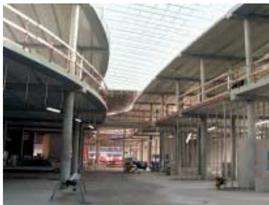
Fig. 10 Customized beams in various designs have been used for the new Saxo Bank building north of Copenhagen. The image shows an edge beam with a round-shaped end.
