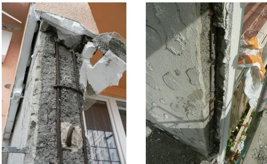
Figure 1. Failure of thermal insulation and concrete cover due to steel corrosion.
